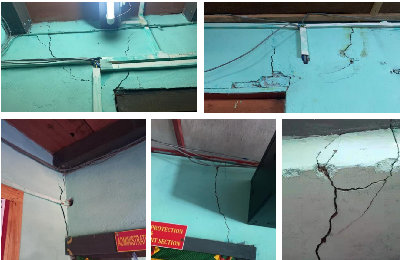
Figure 5: Internal walls of Divisional Head Office (The walls were cracked during 2004 and 2009 earth quake)
